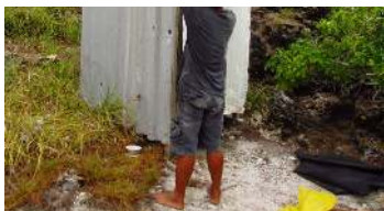
Fixing the outdoor shower at Middle Camp © SIF
