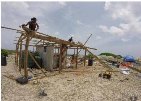
Working on the field camp hut at Cinq Cases © SIF
