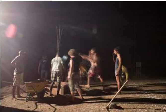
Installation started on the night of arrival! © SIF
