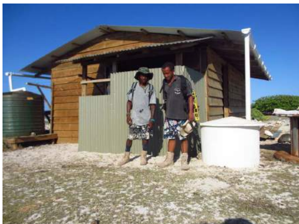
Completed hut © SIF
