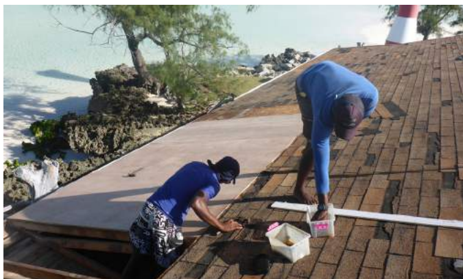
Renovations with a view! © SIF
