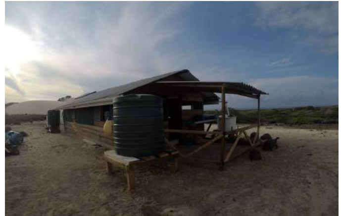
The camp at Dune Jean-Louis has had a new water tank installed and the roof extended © SIF
