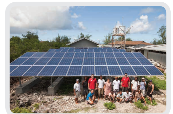
The final solar panel installation and the team that made it happen (R Baxter)
