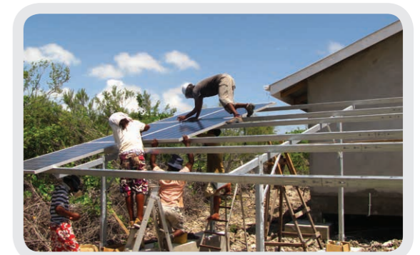
The team install the solar panels (C Quanz)
