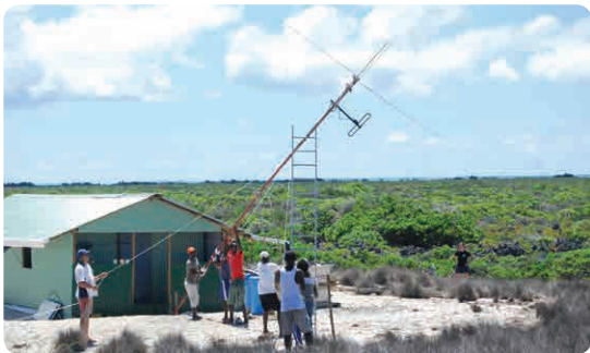
Installing the repeater station at Dune Jean-Louis.
