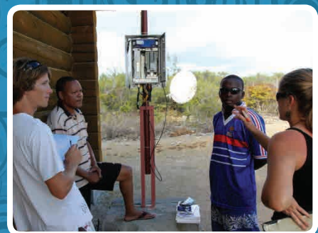
Installation of the new automatic weather station (Dec 2010) (N. Bunbury)
