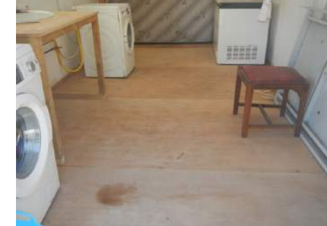
The new wooden floor in the laundry room © SIF
