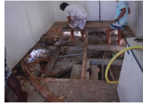
The Aldabra team working hard removing rotten floorboards from the laundry room at the research station © SIF
