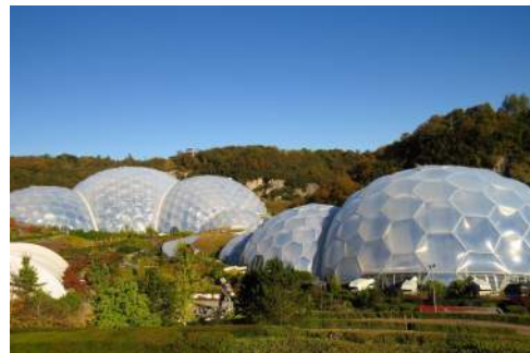
The biomes of the Eden Project in Cornwall, UK © SIF
