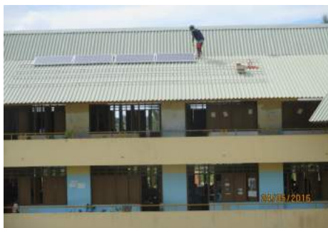
The PV system being installed on the roof of the school © SIF
