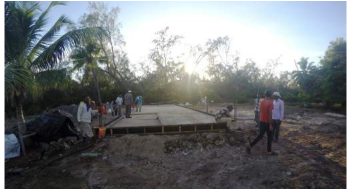
Foundations completed © SIF
