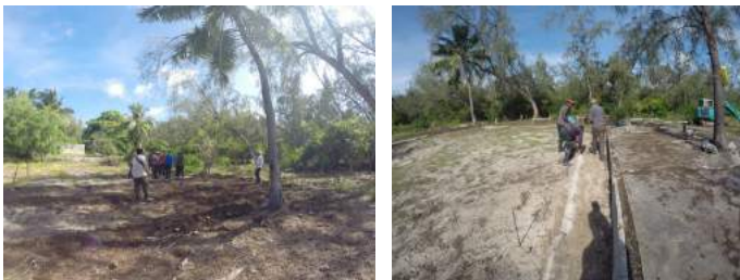
Cyclone shelter construction begins © SIF
