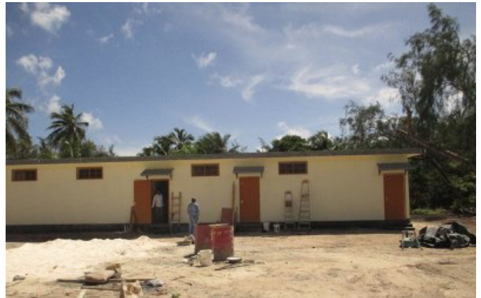
The almost completed shelter © SIF
